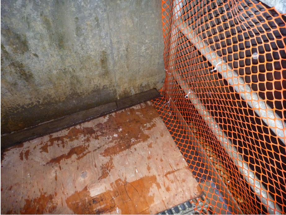
Completed repairs by BON Fisheries
